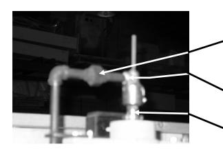
Remove existing 3/8" pipe union and two adjacent pipe nipples between rotary union and 90° elbow on top of machine.
